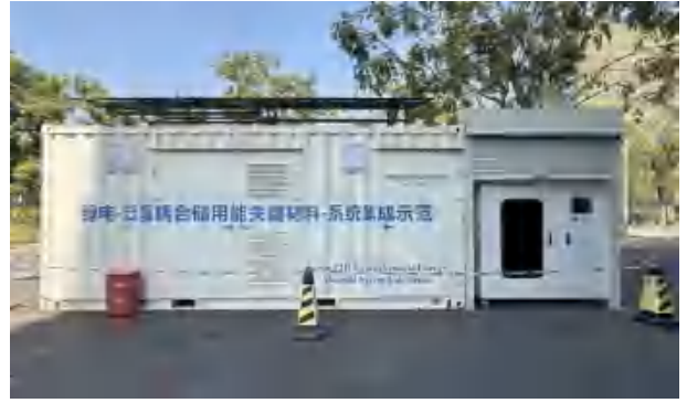
Project: Pan-Hydrogen Coupled Energy Storage Demo Project at a University Scale: 2 Nm 3 /h hydrogen production system, Delivered in 2025 Model: BriLyzer®-M2 PEM Stack
